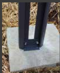
Intermediate profiles fixed on concrete blocks
