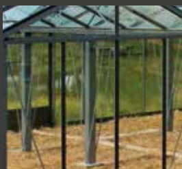
Intermediate profiles fixed on concrete blocks
